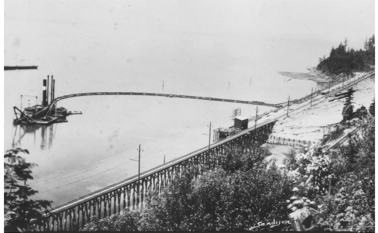
Photo 6. Looking northerly at Clayton Beach area with suction dredge providing fill for platform construction. Photo from Western Washington University, Heritage Resources.
